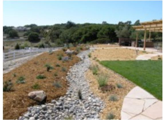
Vegetated swale in Arroyo Grande infiltrates runoff to prevent erosion of the slope below.
