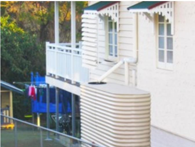
Rainwater from roof is stored in a **cistern** to be used for landscape irrigation.
