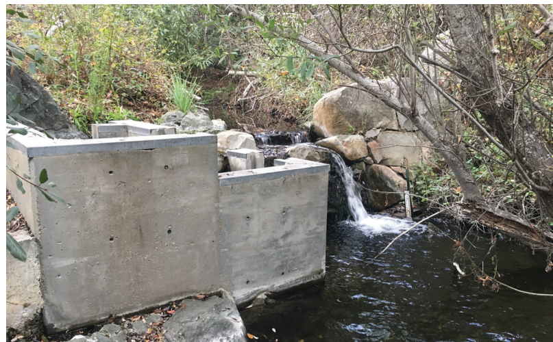
Construction begins next summer to replace this aging concrete passage structure so that fish can access the high quality habitat located upstream.
