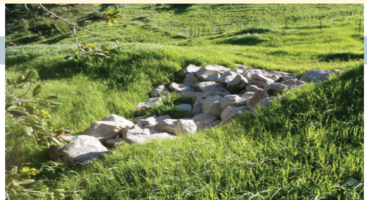
The rocks in this photo provide armoring to prevent rain runoff from causing erosion. This protects both Cal Poly's road and the fish and other wildlife living in nearby creeks.
