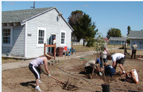
Volunteers help install a greywater system at the Los Padres CA Conservation Corps campus.
