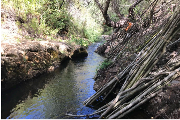
The construction crew lined up Willow stakes along the edge of Chorro Creek before planting them.
