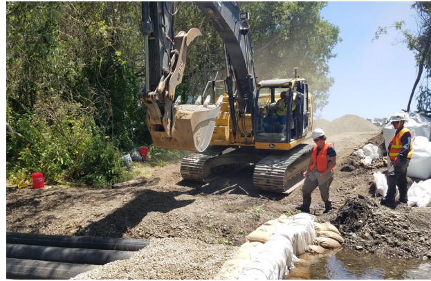
Workers temporarily diverted water from Chorro Creek to protect wildlife during construction.
