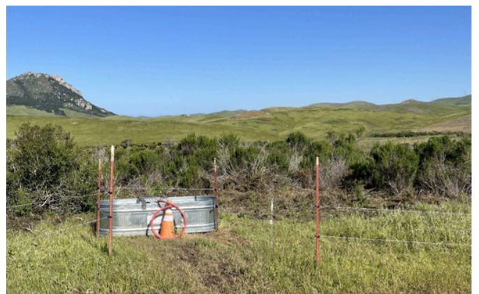
Water stations for grazers are placed on active pastures and fed water via pipes connected to two 5,000-gallon tanks.
